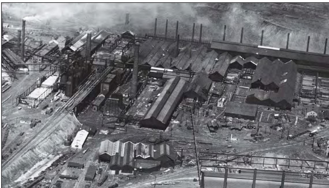
Historic Plate C: Cleveland Steel Works, Grangetown, 1924. Hi-line bottom left with Bessemer furnaces to west of line (Source: Britain from Above website Ref. EPW010144)
