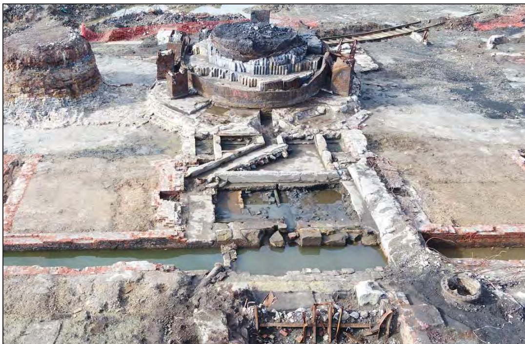
Plate 33: Hoist room for BF4: view north-northwest (Archive Photo Ref. D360)
