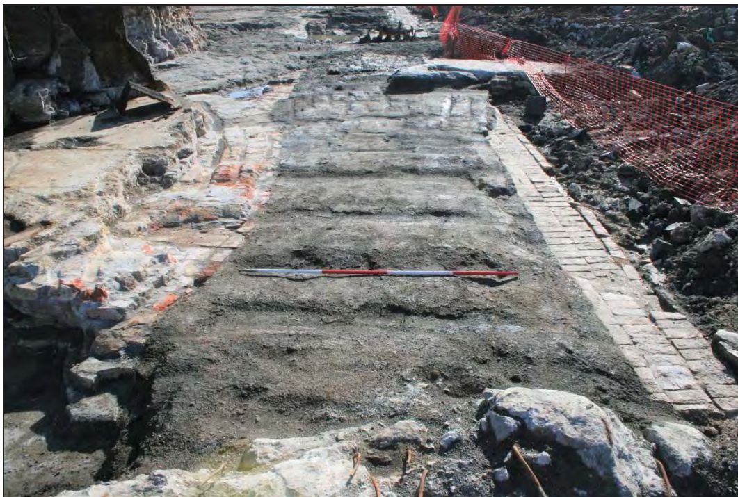
Plate 5: Timber impressions within track bed [26] G8: view south-southeast. 2m scale (Archive Photo Ref. D135)
